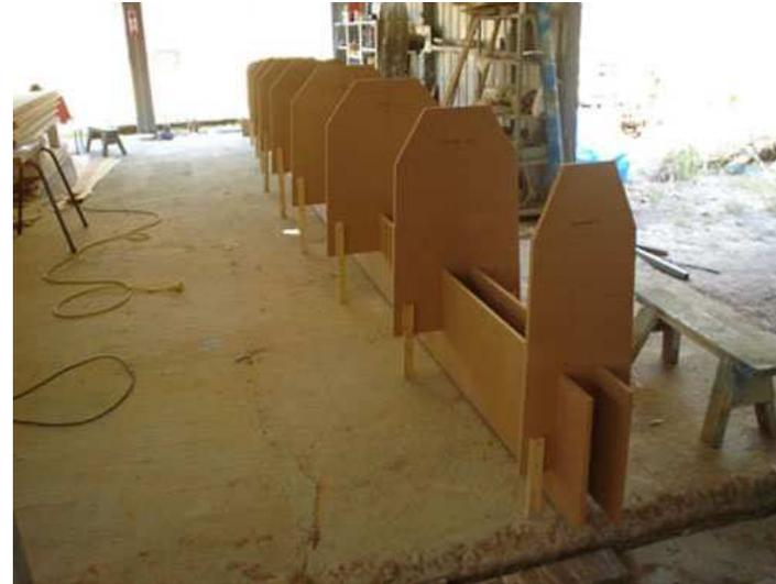
The panels were then attached to the temporary bulkheads using screw (for foam) or wired together (plywood).
