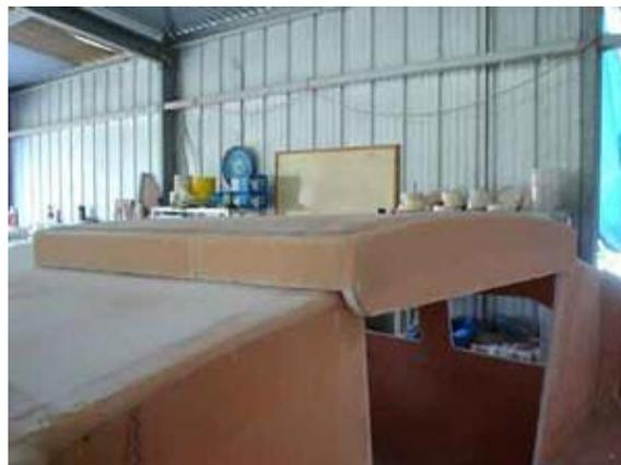
The holes in the cockpit seat risers are cut out when the risers were made. They are taped in and storage divider added. Cockpit seats attached.
